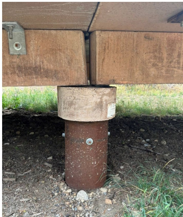
Figure 3. Hollow Steel Pier Footing
