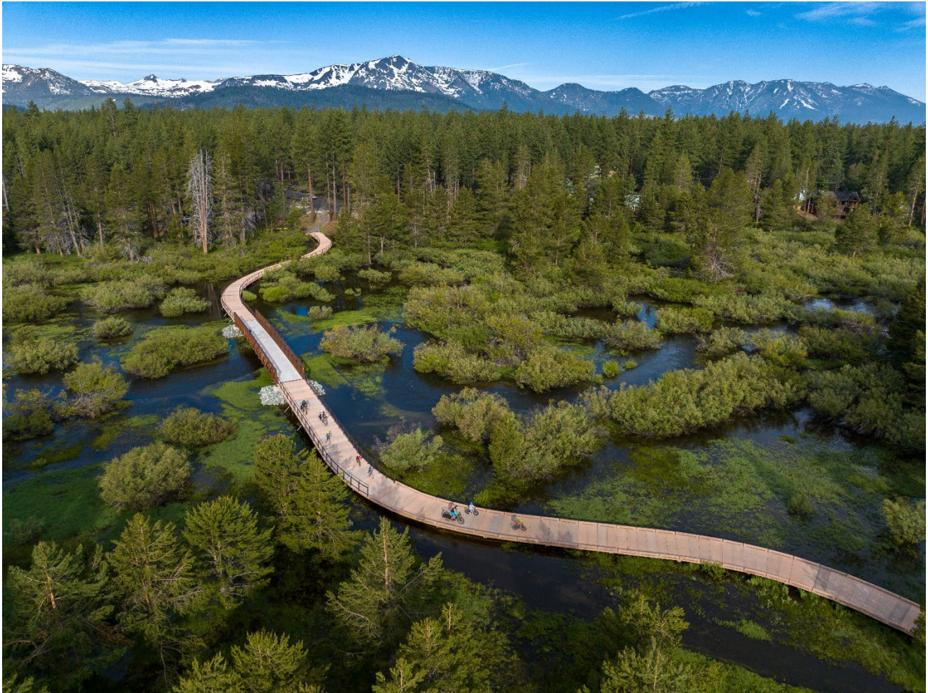
Families riding bicycles to school in June 2023 along the Dennis T. Machida Memorial Greenway, where it crosses Trout Creek in South Lake Tahoe. The Conservancy and its partners designed the trail to use raised crossings to protect wetlands habitat.
