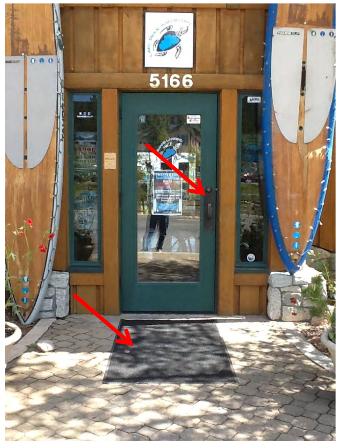
The rug is not firmly attached and the door operating effort requires more than 5 lbs of force.
