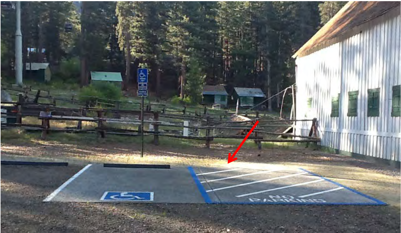
Access path from parking is decomposed granite which has no overall standards to confirm its ability to be firm and slip resistant.
