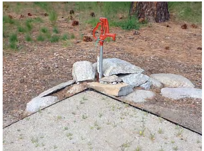
Water spigot location does not provide wheelchair access. Controls exceed 5 lbs. maximum operating pressure and would require tight grasping.
