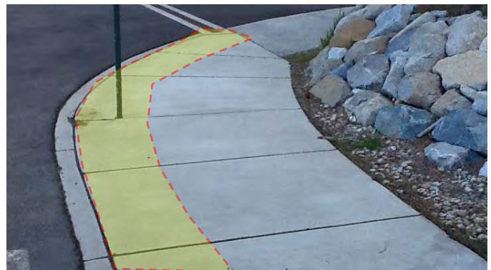
Truncated domes are not provided at flush transitions to vehicular ways.
