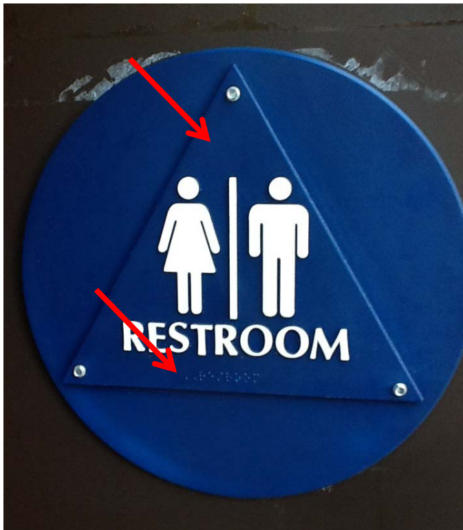
Braille should not be included on door sign and the triangle does not contrast with the circle.
