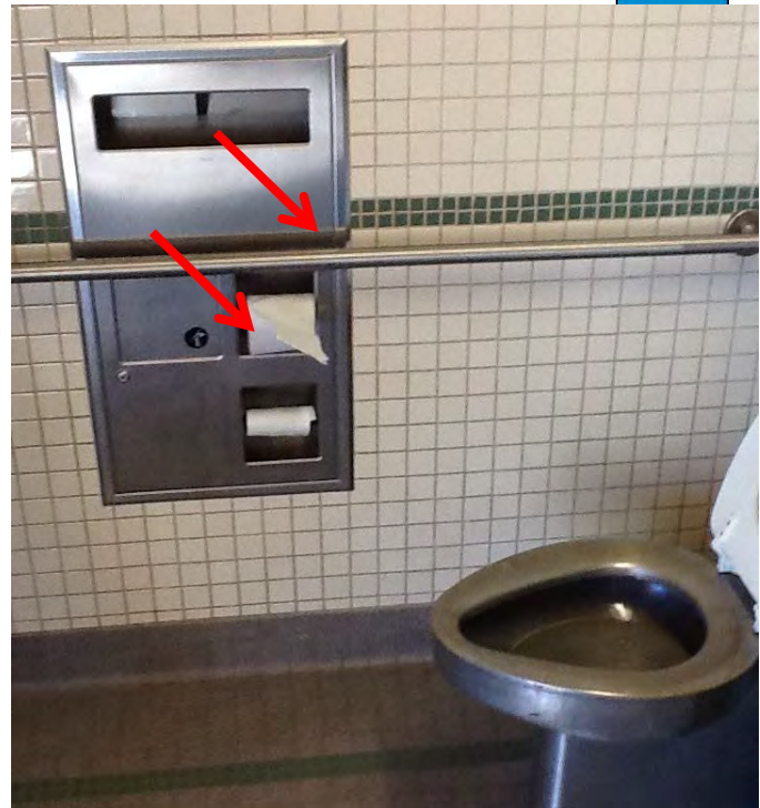
The toilet paper/seat cover dispenser reduces the clear space behind the grab bar to less than 1-1/2". The top roll of toilet paper is not compliant. Should the lower roll be empty, the upper roll would not comply.
