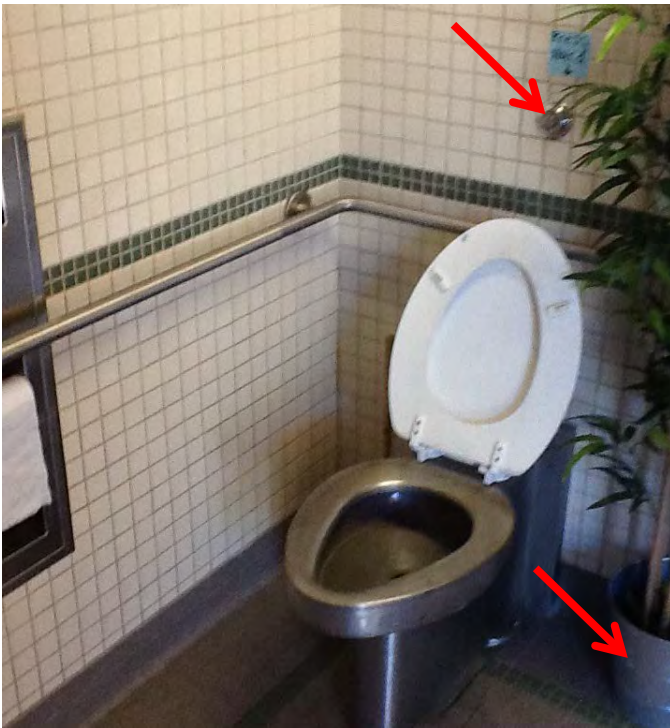
The flush controls are centered on the toilet instead of being located on the fixture's wide side. The potted plant should not be located in the fixture's clear space.
