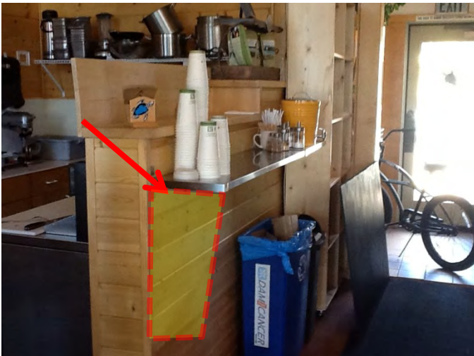
The counter is taller than 34" with no lower accessible portion. An end panel is required down to 27" above finish floor for cane detection. Shelving provides the cane detection on the far end.
