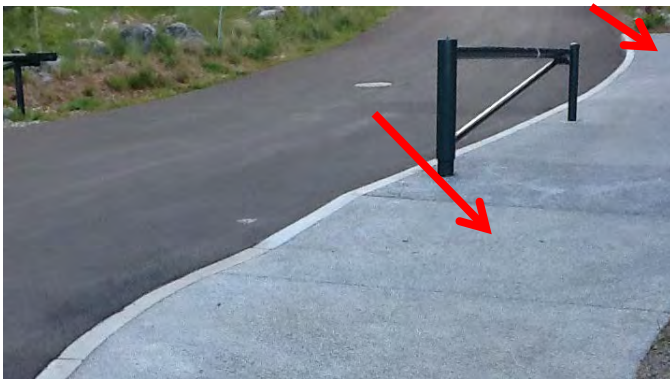
Running slopes exceed 5% and cross slope exceeds 1:48 (2%) in sections.
