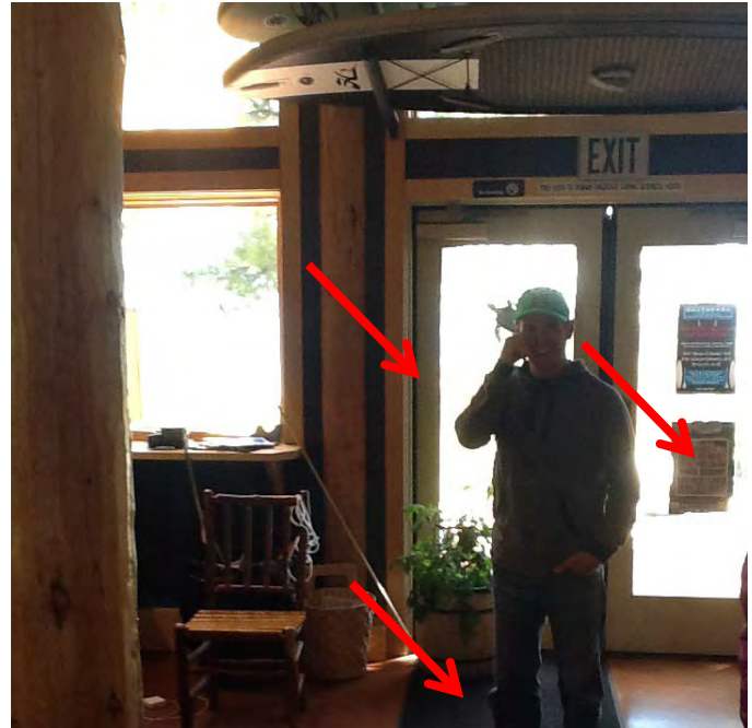
Rug is not firmly attached and no ISA is provided at the entry. A tactile and braille "EXIT" sign should be provided.
