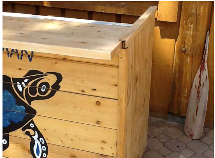
Outdoor counter height is greater than 34" with no lower accessible portion.
