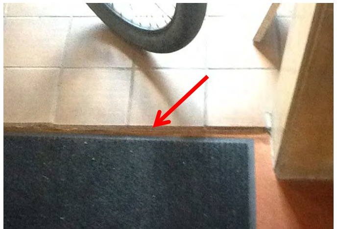
The threshold's vertical change exceeds more than 1/2" overall. Provide a rubber or aluminum transition strip.
