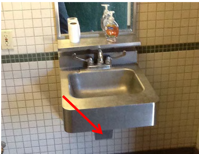
The metal shroud invades the knee space so that the knee clearance does not extend 8" from the front edge of the lavatory.
