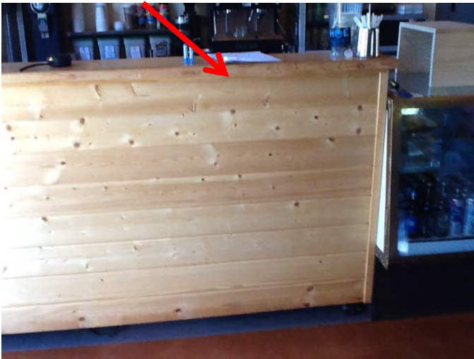
Counter height is greater than 34" with no lower accessible portion.
