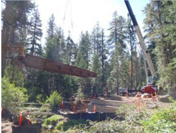
Dollar Creek Shared-Use Trail – During Bridge Construction
