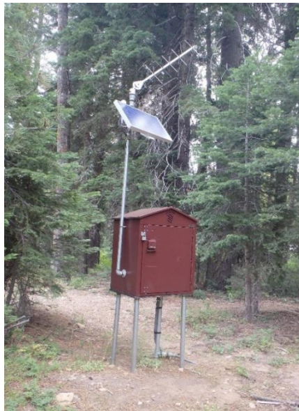
Stream gaging structure
