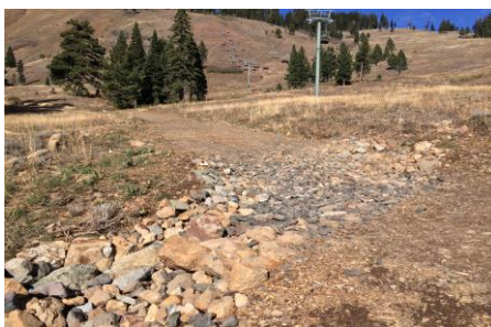
Sherwood Ski Lift access road post treatment
