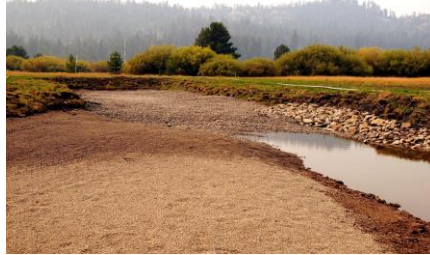
Sunset Stables Reach 5 Construction 2013
