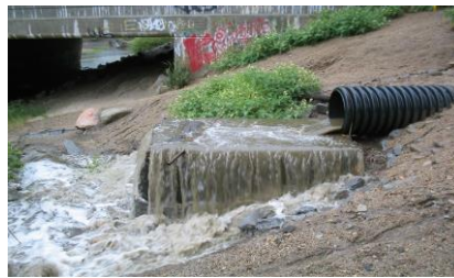
Sierra Tract stormwater runoff (pre-project)
