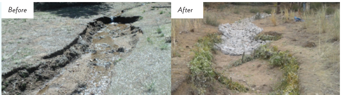
Stream channel enhancement projects improve lake clarity by reducing sediment caused by eroding stream banks.
