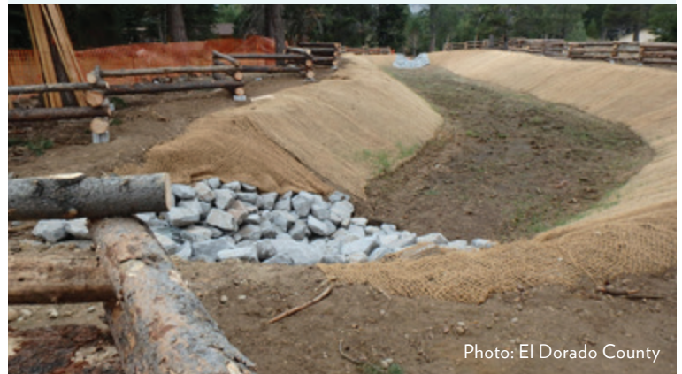
This infiltration basin will clean storm water by allowing it to filter into the ground before heading to Lake Tahoe.
